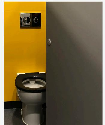
our manufacturing facility so that T-IPS could install each unit 50% faster than plain panel alternatives. The access panels were mounted onto linear-bearing hinges so that access to concealed duct space could be gained quickly without having to manually remove panels.
